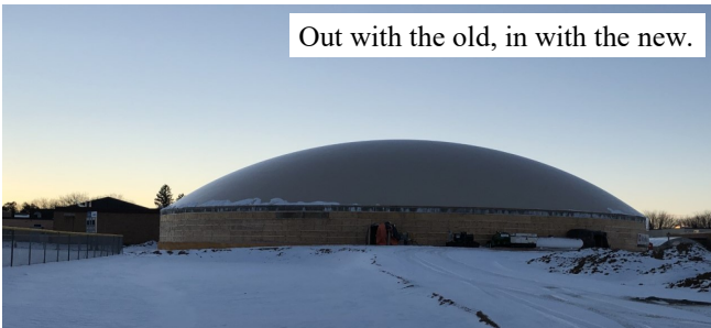
The peak of the R. J. Tack Auditorium looms to the west and south, overseeing construction of the Rockets new home in the Dome.
